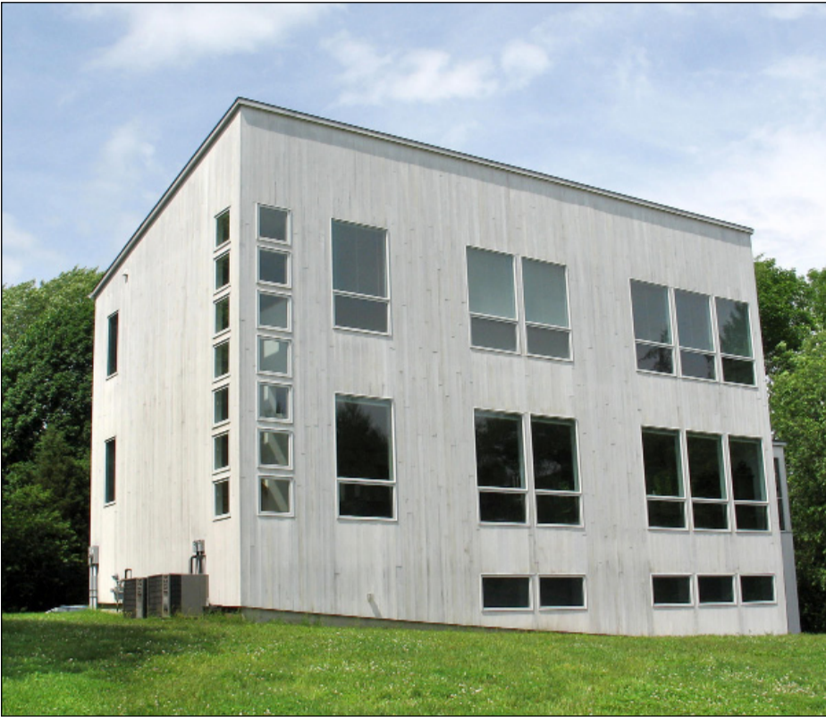
Completed in 2002, the house features vertical siding of white-stained cedar and banks of windows on its exterior. The interior combines white walls with pale birch floors and black granite countertops.
